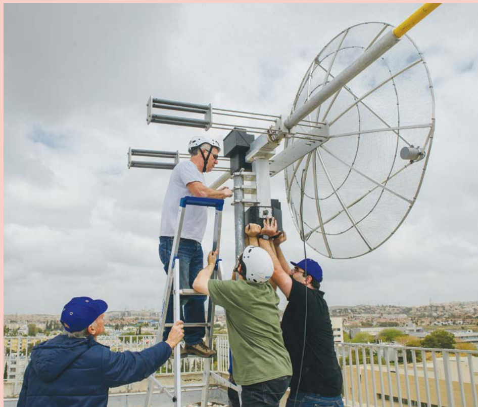
↓ Installation of BGU's Satellite Ground-Receiving Station
